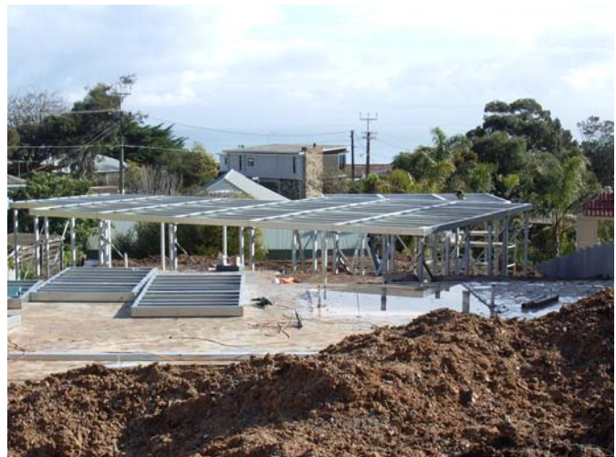
Figure 3: Supafloor platform being erected
