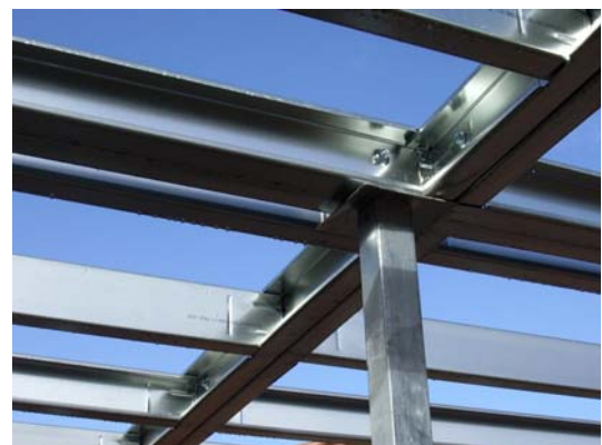
Figure 5: Supafloor over column support
