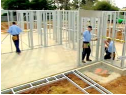
Figure 4: Walls being erected
